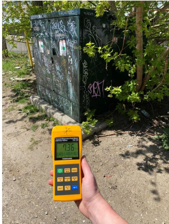
Figure 3: Elevated A.C. magnetic field readings recorded beside existing transformer.
